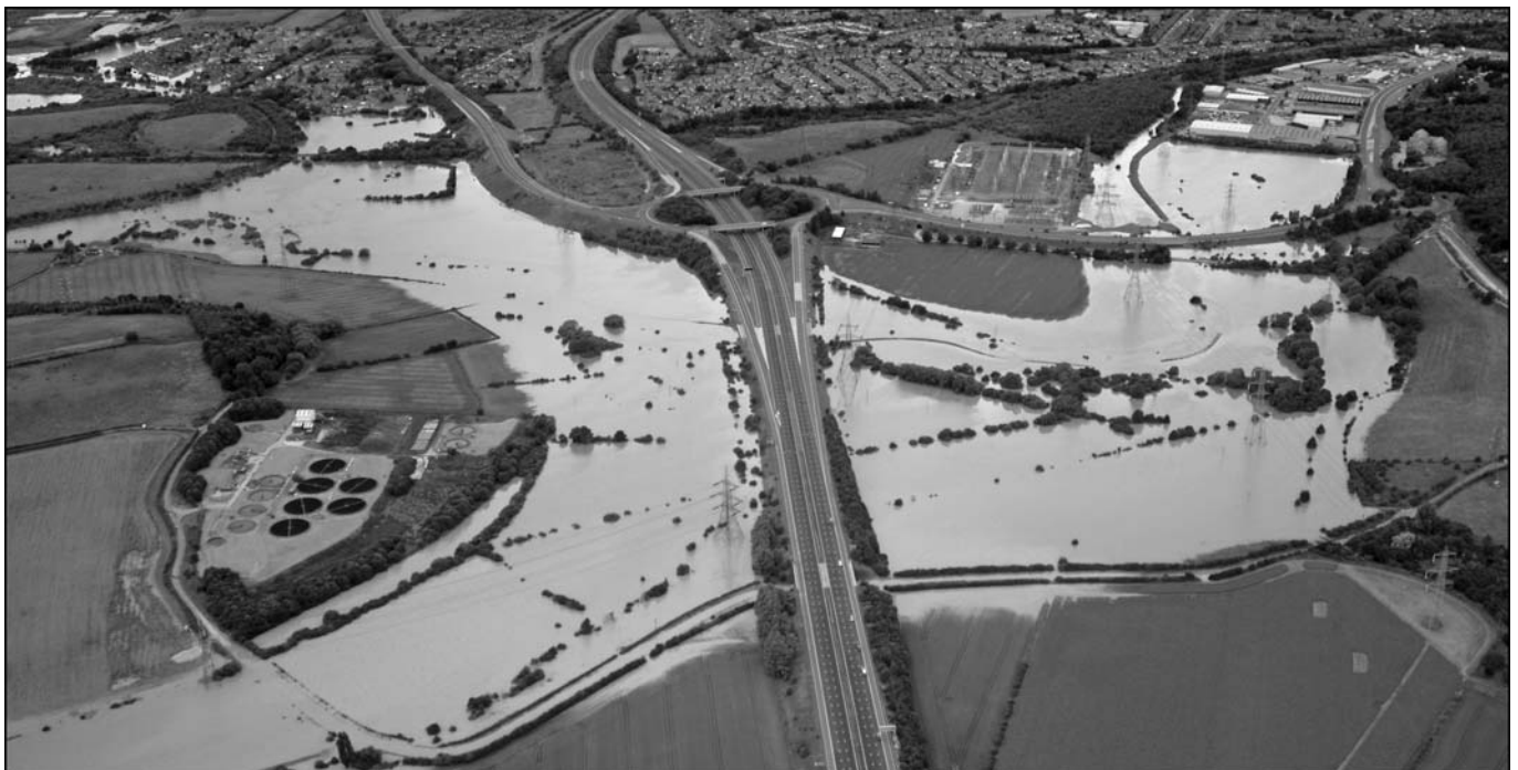
Active floodplain of the River Rother, with backflooding into Catcliffe village (top left), beneath junction 33 on the M1.
