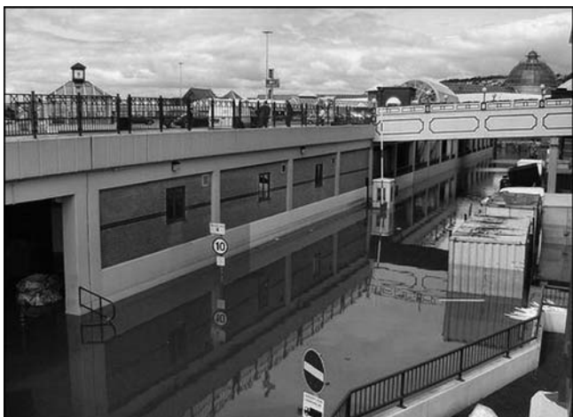
Floodwater in the Meadowhall Centre.
