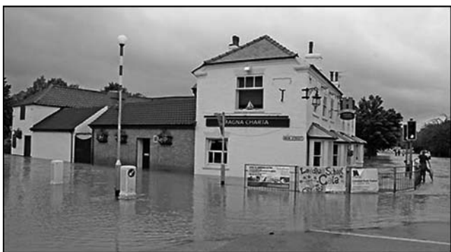
The Magna Charta public house in Lowdham, flooded on June 25th (photo: James Brunton).
